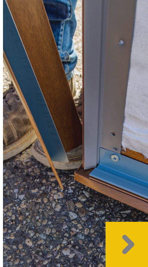
Align bottom corner of two piece corner cap to bottom of base flashing.
