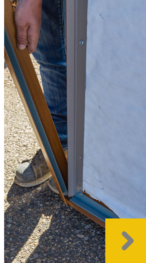
Start to press the corner cap in on bottom corner.
