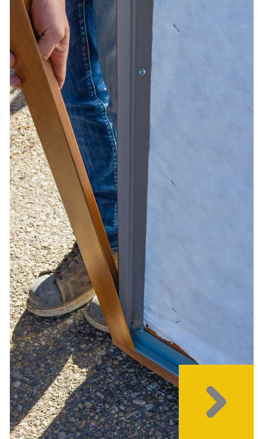
Working your way up corner cap continue to snap in place.
