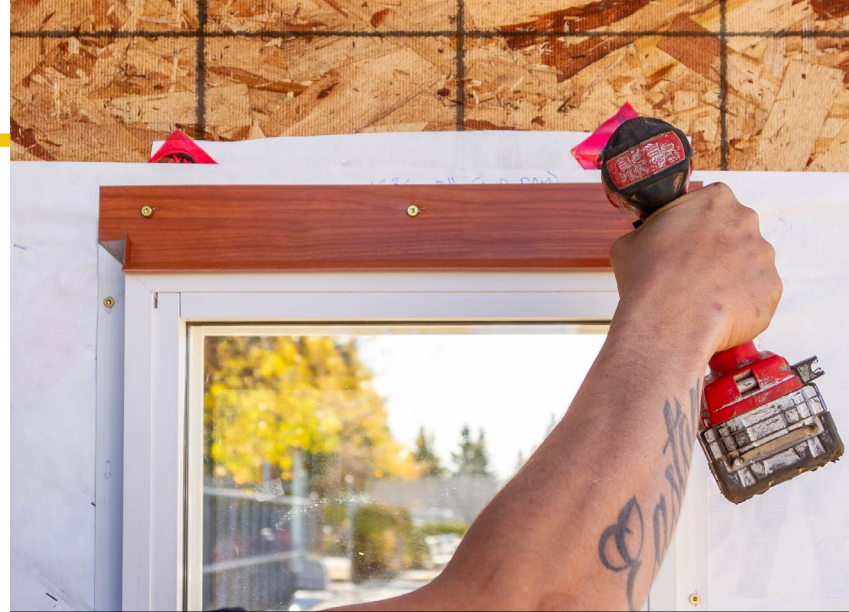
SECURE THE DRIP FLASHING
