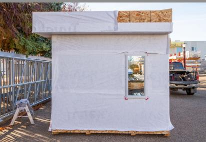
Prior to the installation of InterClad, ensure that a water-resistive barrier is installed correctly to the manufacturers' instructions.
