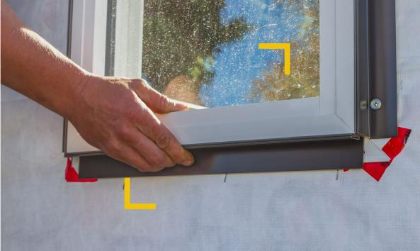
Align Lower window flashing (2 piece base) with frame. Fasten the 2 piece base in place. Align Upper window flashing with top of the side window flashing. Secure in place.
