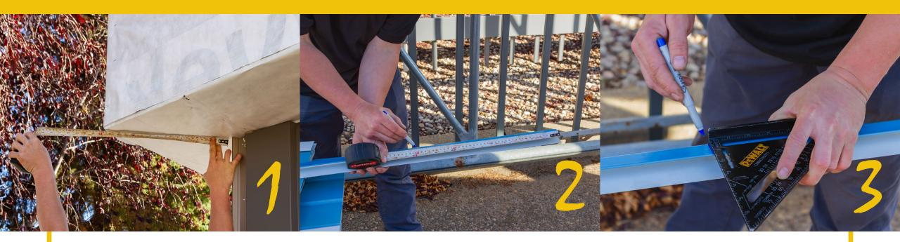
**1. Measure** from corner of wall to the outside corner for the soffit.
