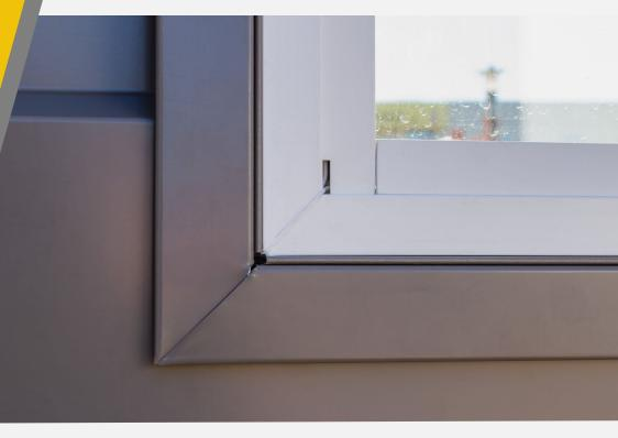
Mitre both sides of the upper cap flashing and snap in place . The hem of the upper window cap flashing will need to be opened up so it can slide over the side cap flashings.
