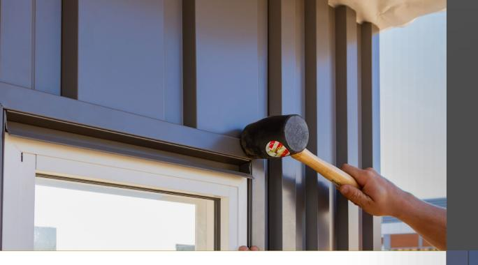
**Measure** the length of the window and add 2" to the length of the cap.
