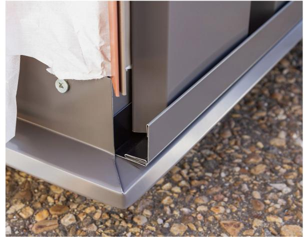
**Push** the 2-piece J-trim top into its base. Then using a rubber mallet tap it tight into the lock.
