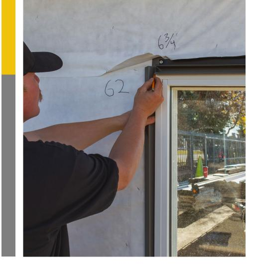
The base should align with bottom of the window and the top of the end dam. Secure in place with a pancake screw.
