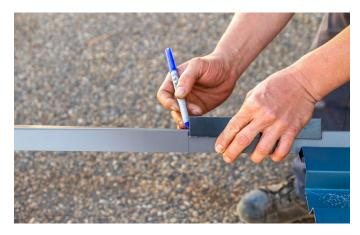
After installing the upper and lower two-piece base flashing, measure the distance for the panel that needs to be notched out for the bottom of the window.
