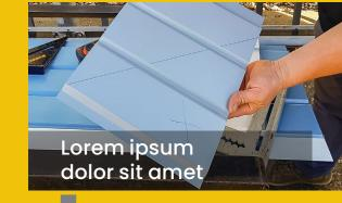
Draw a line from these two points and cut the panels along this line. INTERCLAD
