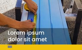
To start, lock together enough panels to cover the mitre section that are precut to the soffit depth.
