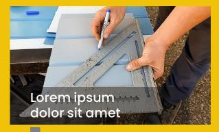
Markout edge of the wall panel from the previous step and mark the corner of the the soffit.
