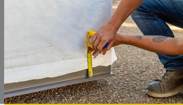
Measure the length from the drip flashing. Cut, using snips or a cold cut saw blade. Never use abrasive cut off wheels with metal flashing.
